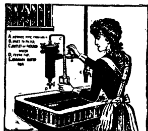
This illustration shows FILTER (H), fitted to Ordinary Household Service pipe over sink; the cost of which is 30/- only, Complete.
