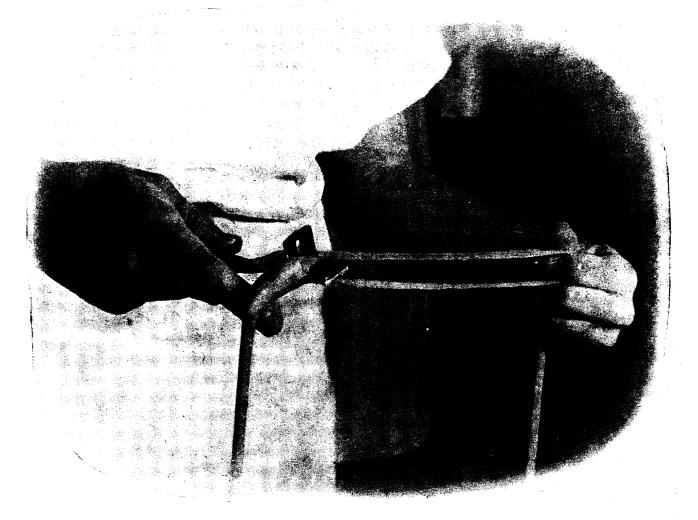
Manufacturing LHC. Stage 1. After thawing, New Zealand milk lamb intestines are split into three ribbons to facilitate subsequent treatment.
