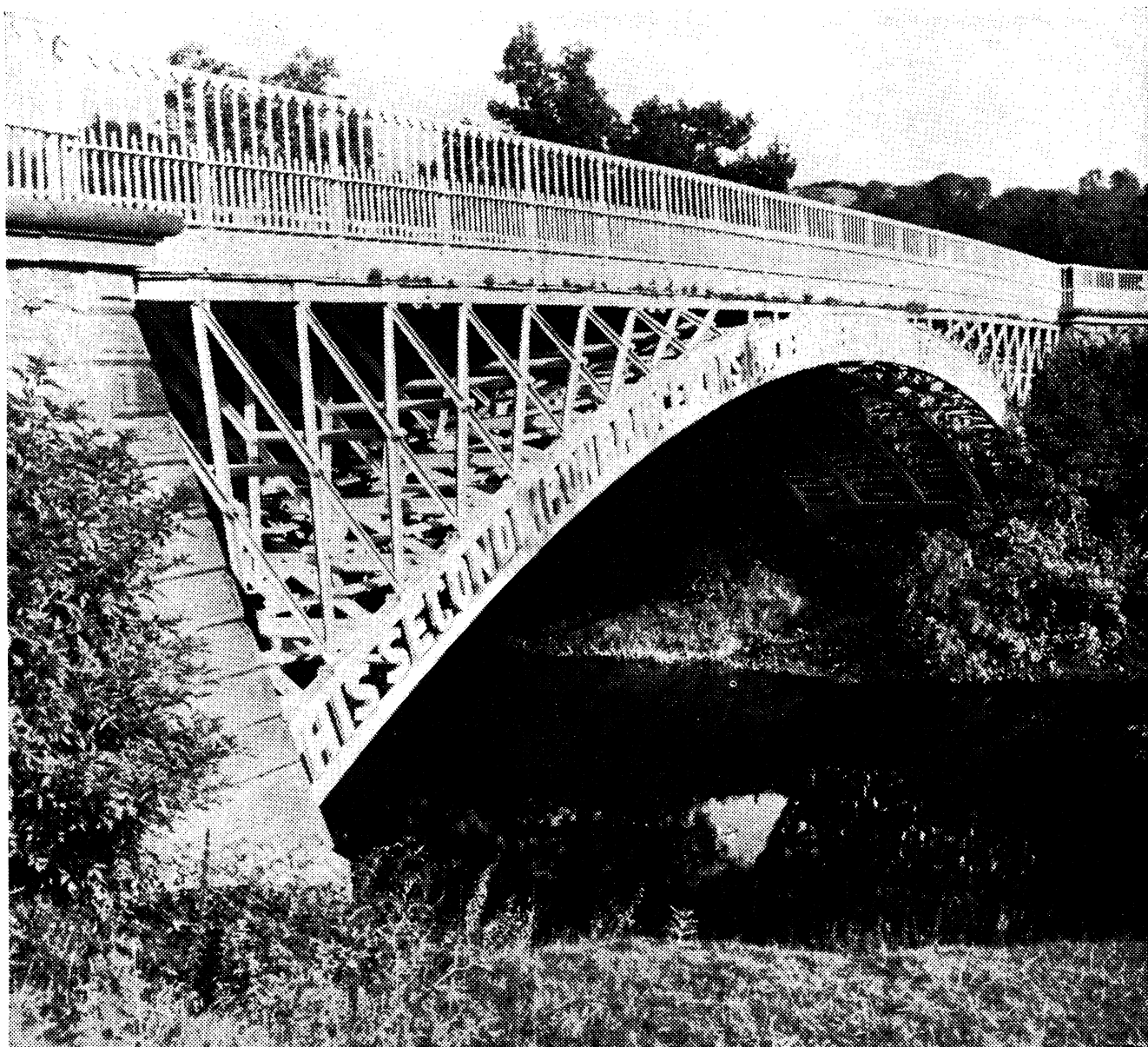
This cast-iron bridge was erected in 1852 at Abermule in Montgomeryshire over the Severn.
