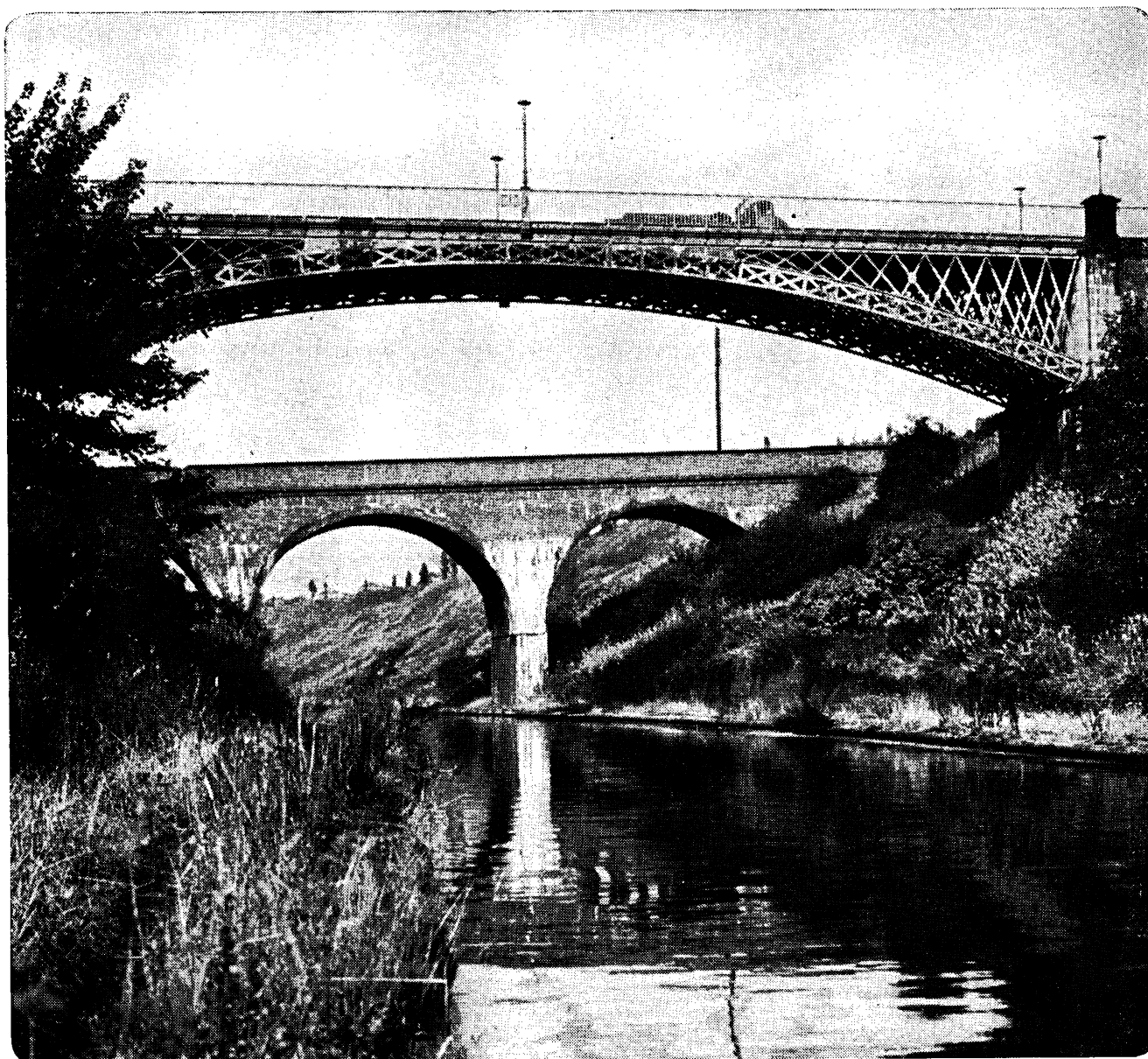
The cast-iron Galton Bridge at Smethwick was designed by Thomas Telford, and built in 1829. It carries the road over the Birmingham Canal.
