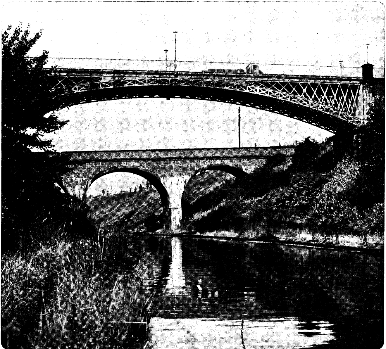
The cast-iron Gallton Bridge at Smethwick was designed by Thomas Telford, and built in 1829. It carries the road over the Birmingham Canal.
