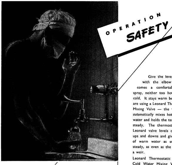
Give the lever a nudge with the elbow and out comes a comfortably warm spray, neither too hot nor too cold. It stays warm because you are using a Leonard Thermostatic Mixing Valve — the valve that automatically mixes hot and cold water and holds the temperature steady. The thermostat in the Leonard valve levels off all the ups and downs and gives a flow of warm water as smooth, as steady, as even as the tide over a weir.
